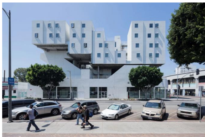
Figura 1: Fachada do Star Apartments, Los Angeles
